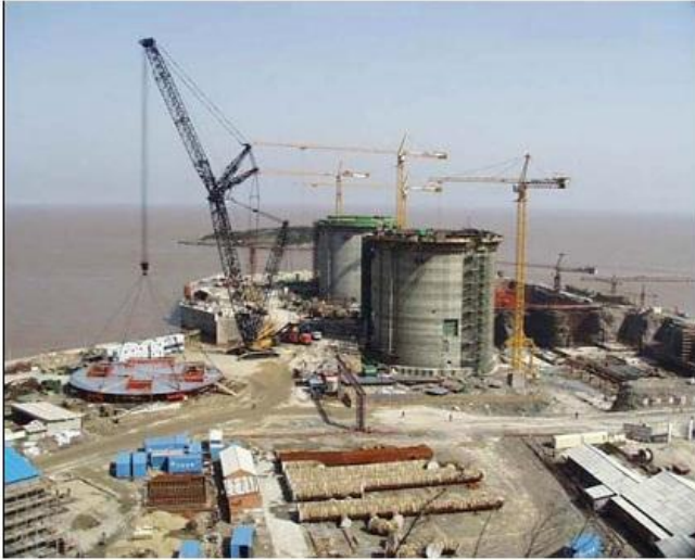
Very Heavy Lift Crane At Qinshan, China
