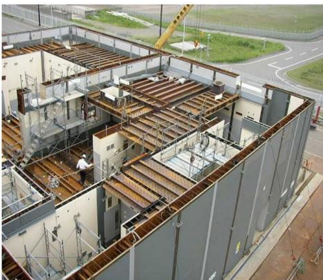
Steel Plate Reinforced Concrete
