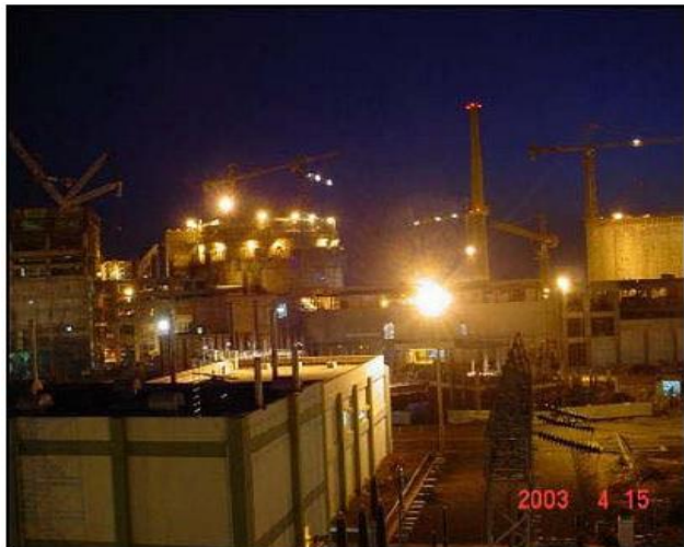
Night View Of Site Activities At Tarapur , India:
