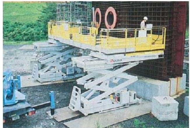
An Automatic Scaffold And Horizontal Rebar Feeding Machine At Kashiwazaki Kariwa-6 In Japan:
