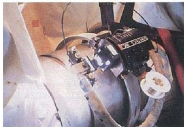
Automatic Piping Welding At Kashiwazaki Kariwa-7 in Japan
